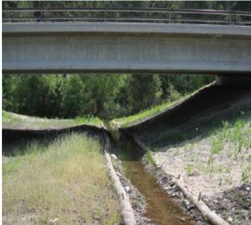
Figuur 7.6: Viaduct state route 40, Florida, USA, foto Marcel Huijser
