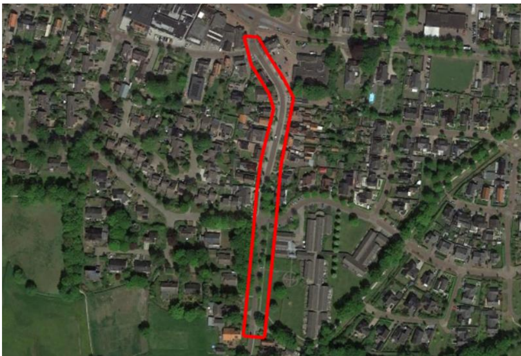
Figuur 76: Julianaweg (bron: Google Earth)
